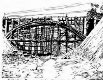
Erecting Formwork for Park Row Bridge, 1941
