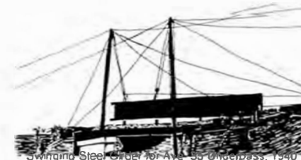
Swinging Steel Girder for Ave. 33 Underpass, 1940
